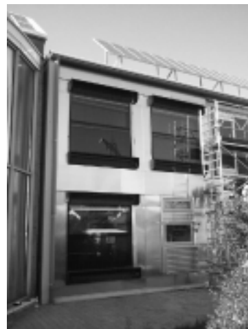
Fig. 1. View of the FASTEST site in Freiburg, showing four facade elements
